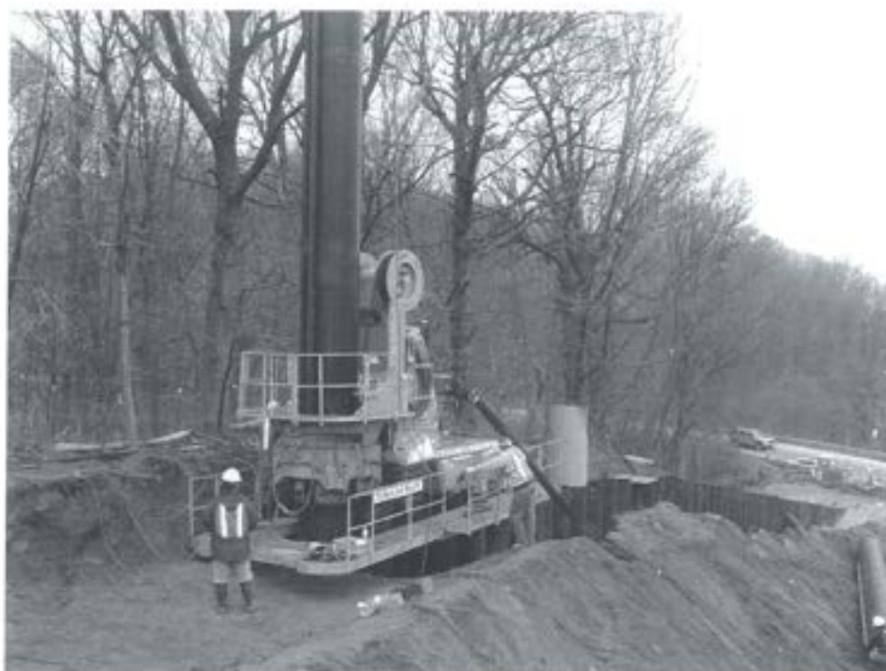
Figure 1. A row of 914 mm diameter tubular piles being installed by a press-in piler (New York, USA).
